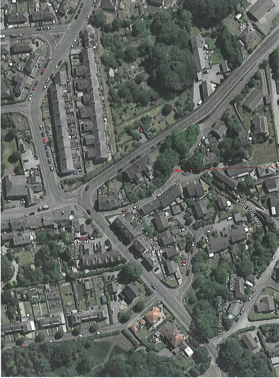
Tree Location. Car park on Skinner Street, Cockermouth.
